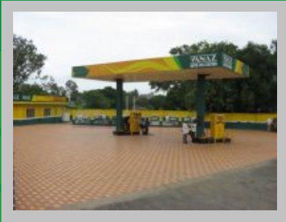
VANAZ LPG STATION, Pune ▲
